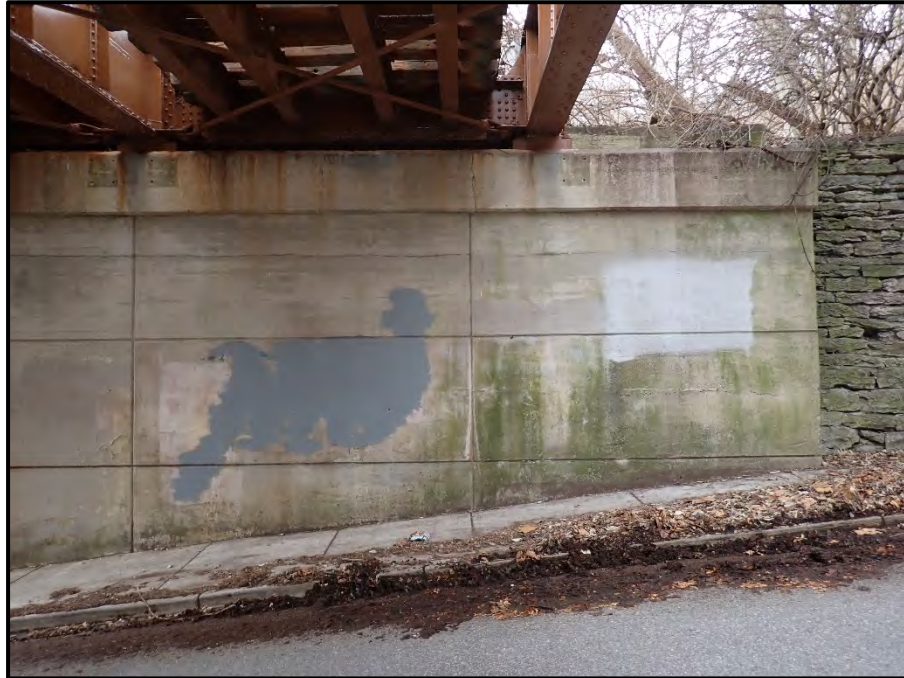
Photo 7 – Looking west at the west abutment. Note: minor algae growth on the bottom half of the abutment wall under girder 1.
