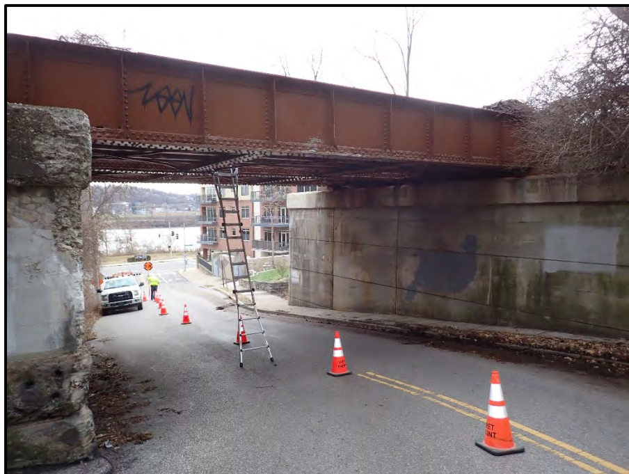
Photo 2 – Elevation looking southwest.
