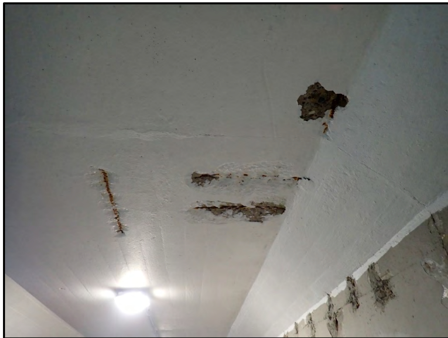
Photo 11 – Looking northwest at 30 SF of intermittent spalling on the west wall, up to 1" deep.
