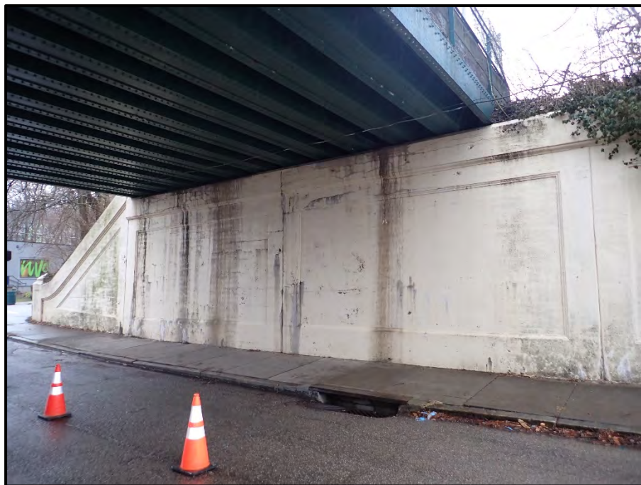
Photo 6 – Looking northeast at the east abutment elevation.
