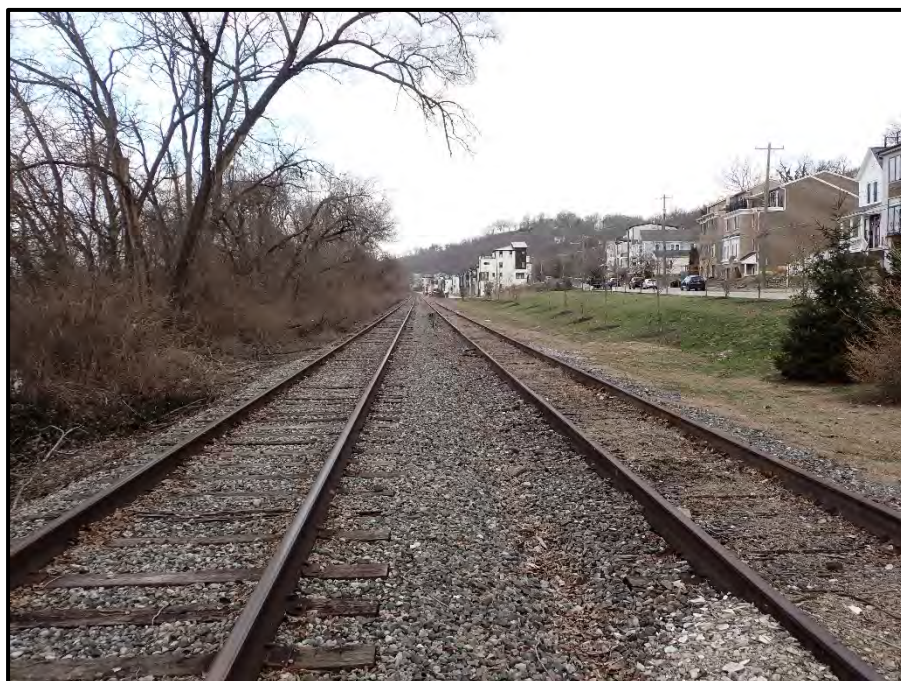
Photo 4 – Top of rail over tunnel, looking west.
