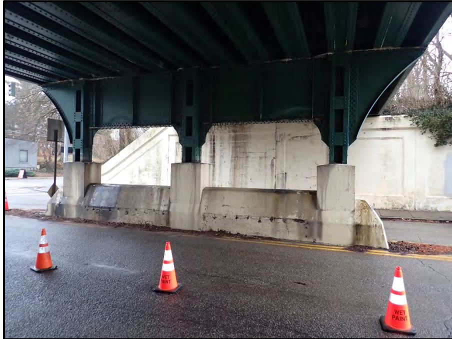
Photo 7 – Looking west at the overall of the west face of pier 1.
