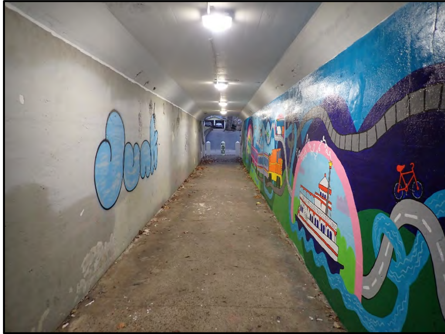
Photo 5 – Looking south at the typical inside of tunnel condition.
