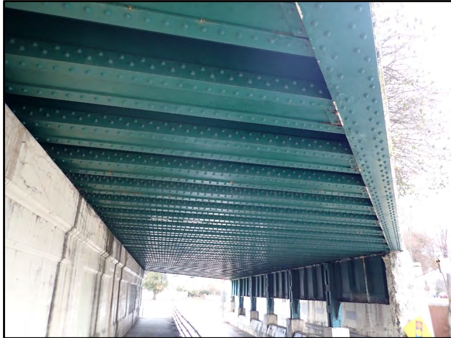
Photo 5 – Looking south at the general underside condition of span 2.
