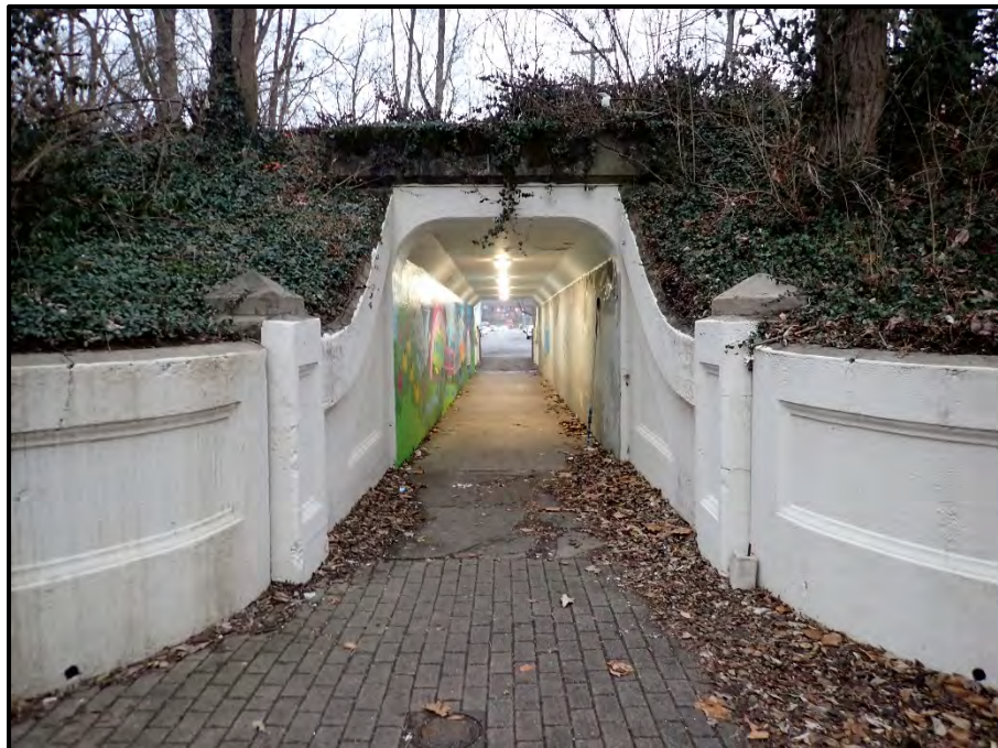
Photo 2 – Elevation looking south.
