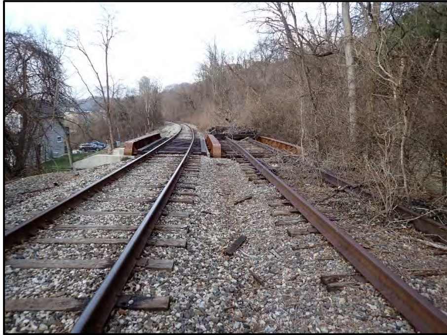
Photo 3 – End view looking west.
