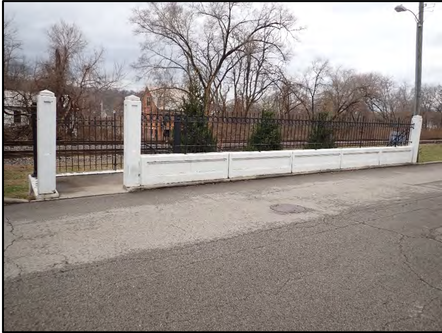
Photo 9 – Looking south at the overall of the above ground portion of the retaining wall from Walworth Ave.
