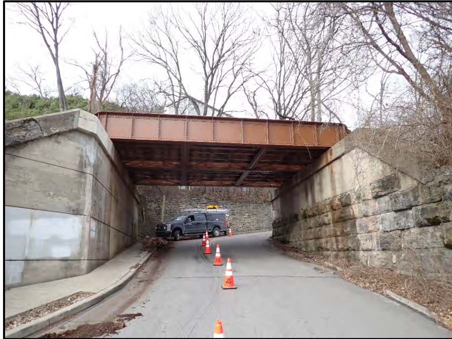
Photo 1 – Elevation looking north.
