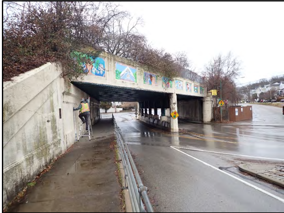
Photo 1 – Elevation looking south.
