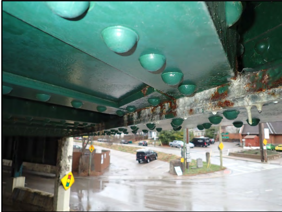
Photo 9 – Looking northwest at the typical efflorescence and water staining on the bottom flange of beam 3 at the north girder in span 2.
