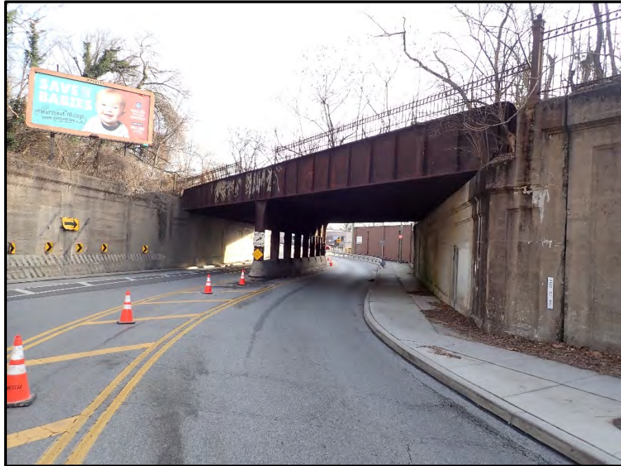
Photo 1 – Elevation looking south.
