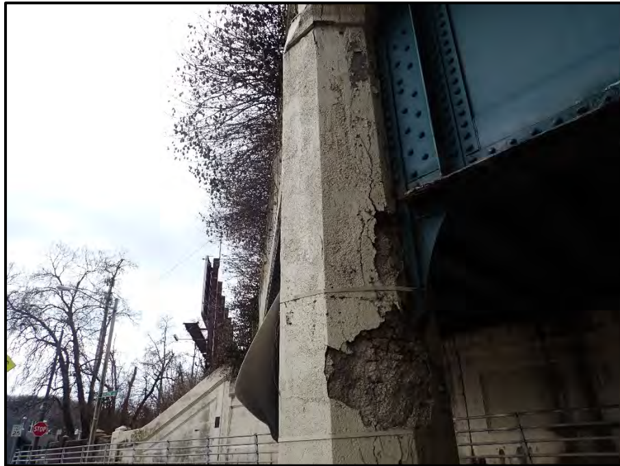
Photo 16 – Overall, of north column (column 1). Note: column is in similar condition to column 7. Steel frame is not exposed.
