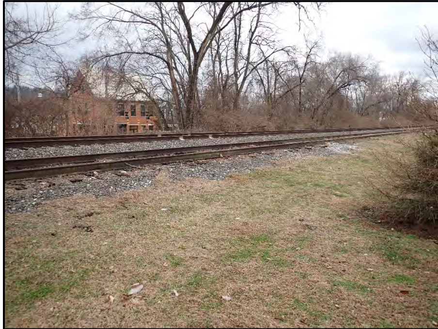
Photo 7 – Looking southwest at the typical top of track over tunnel condition.
