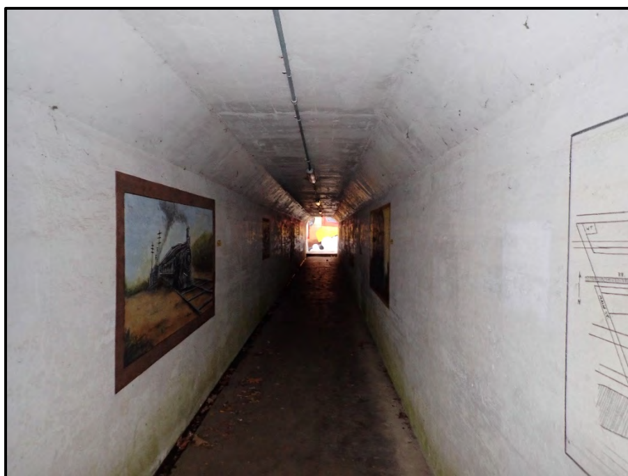
Photo 6 – Looking north at the typical inside of tunnel condition.
