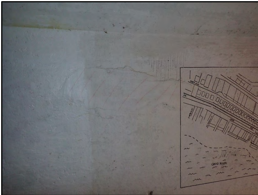
Photo 10 – Looking west at 3' x 1' unsound patch on the west wall 5' from the north end of the tunnel.
