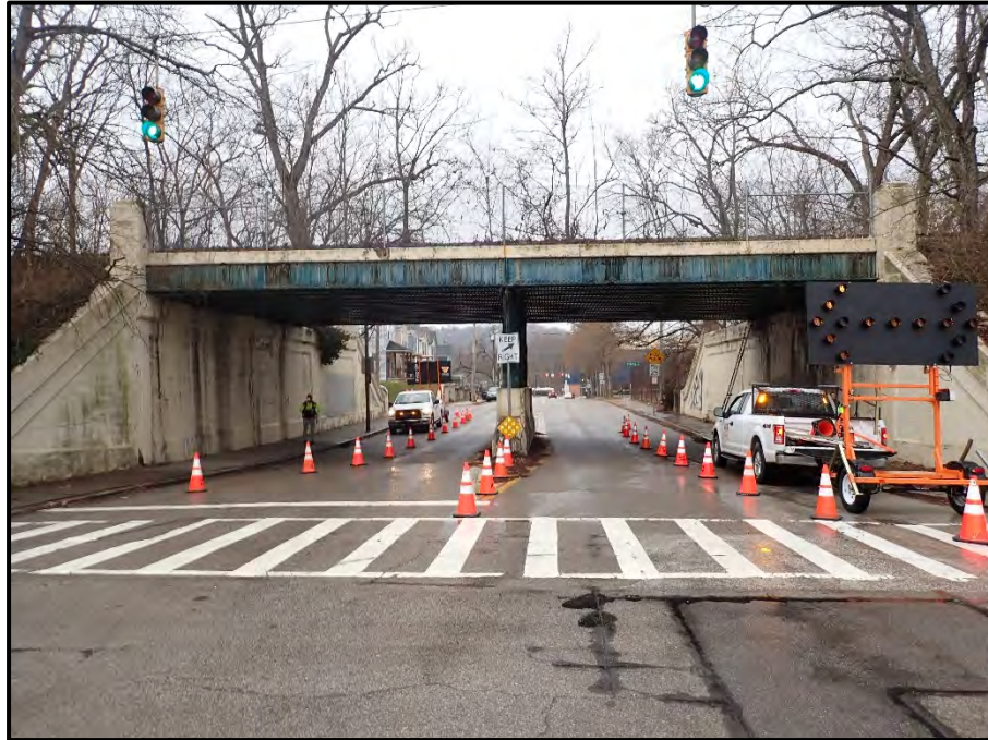
Photo 1 – Elevation looking south.
