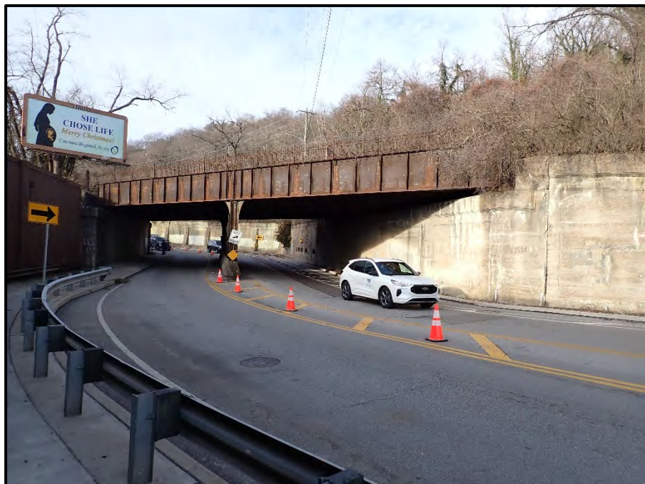
Photo 2 – Elevation looking north.
