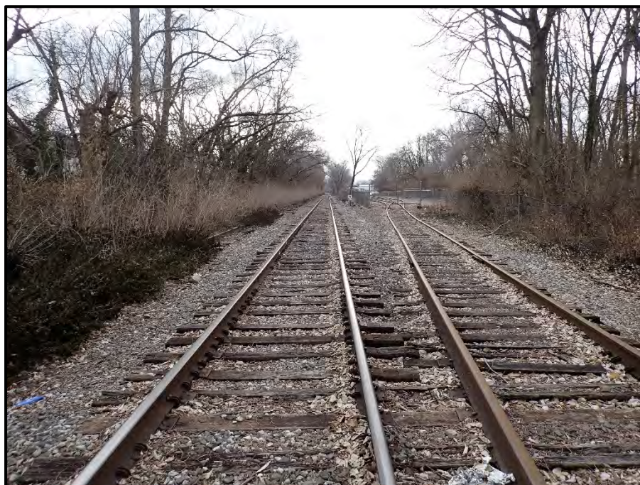
Photo 3 – Top of rail over tunnel, looking east.
