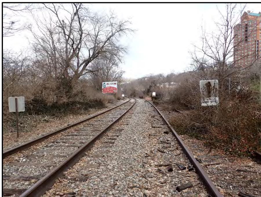
Photo 3 – End view looking west.
