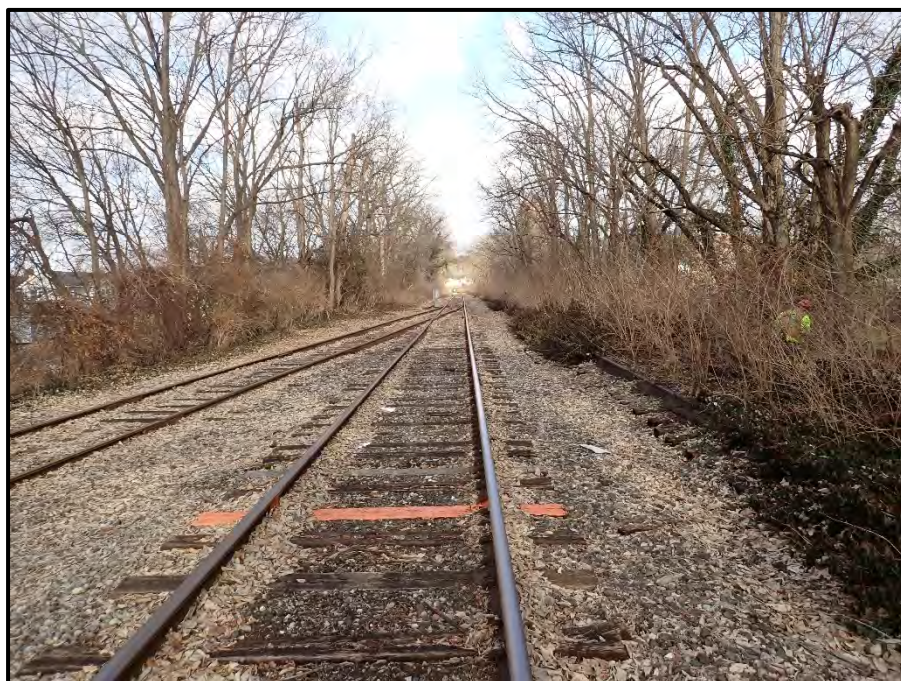
Photo 4 – Top of rail over tunnel, looking west.
