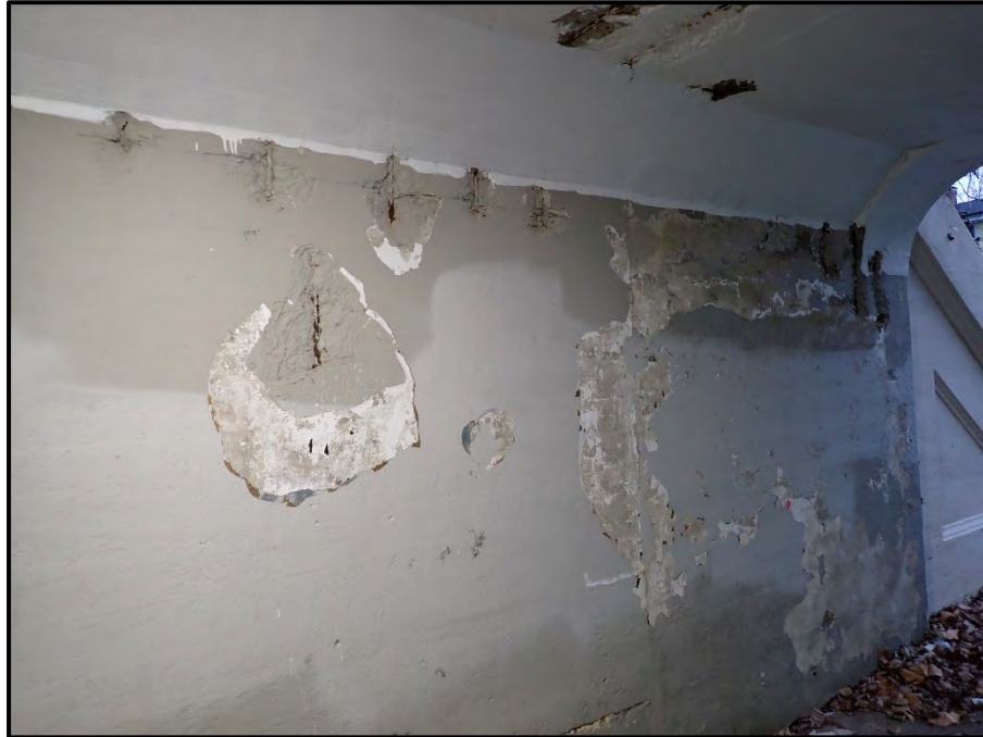
Photo 11 – Looking northwest at 30 SF of intermittent spalling on the west wall, up to 1" deep.
