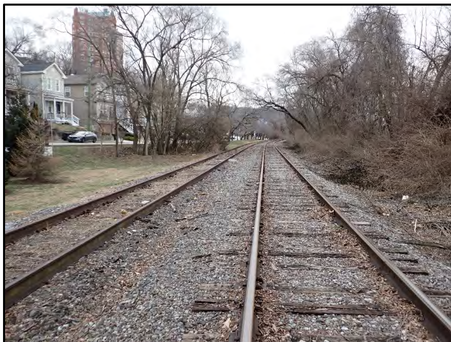
Photo 3 – Top of rail over tunnel, looking east.
