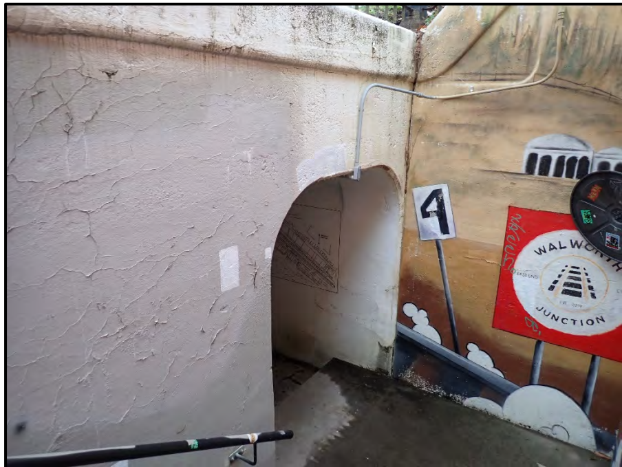
Photo 2 – Elevation looking southwest.
