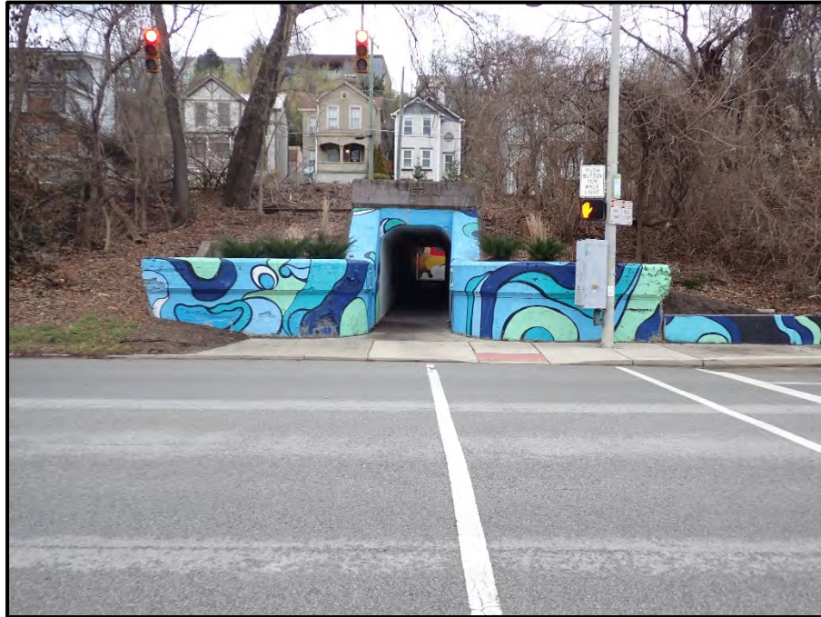
Photo 1 – Elevation looking north.
