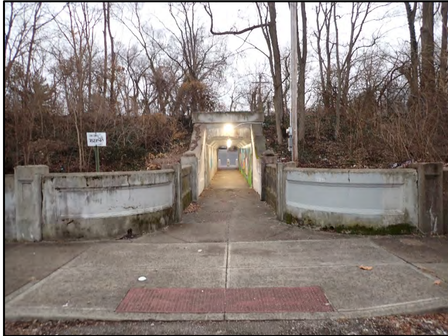
Photo 1 – Elevation looking north.
