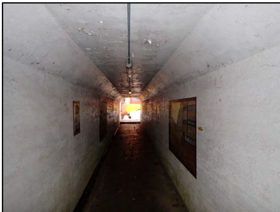
Photo 5 – Looking north at the typical inside of tunnel condition.
