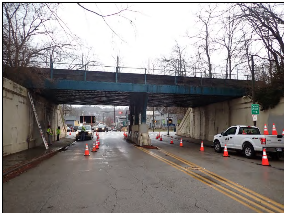
Photo 2 – Elevation looking north.
