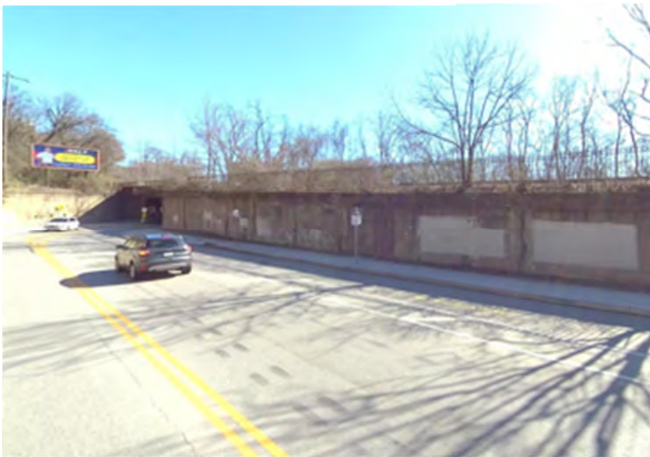
Figure 13 – Existing Retaining Wall
