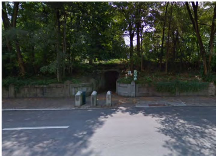
Figure 46 – Congress Avenue Tunnel
