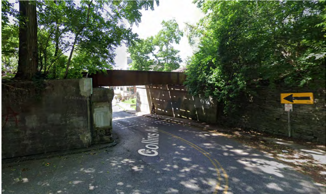
Figure 22 – Collins Avenue Bridge
