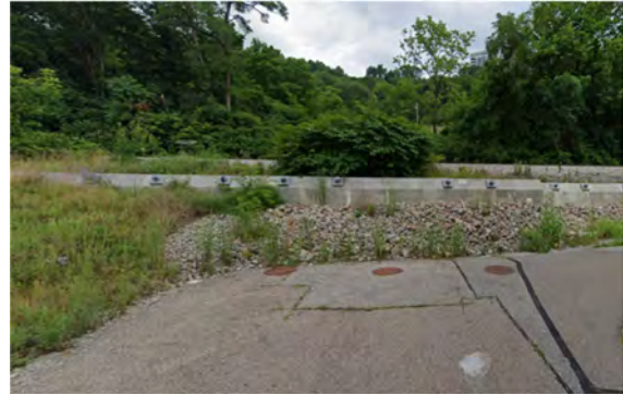
Figure 19 – Existing Tie-Back Wall
